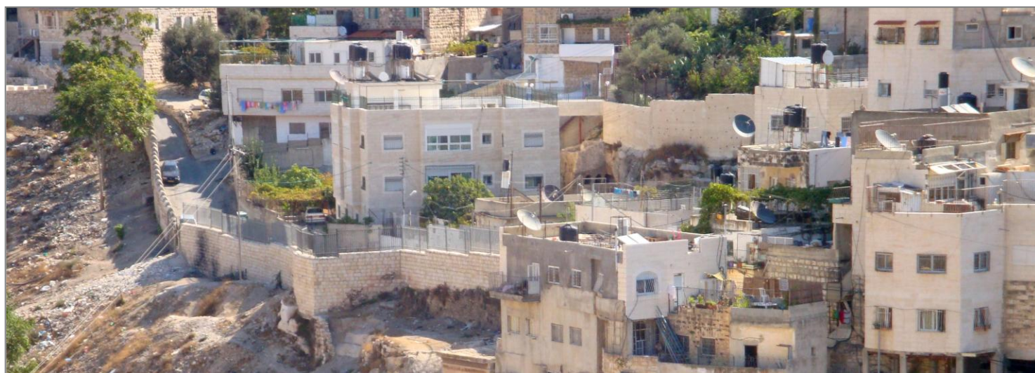
Photo of the mainly Muslim populated Silwan neighborhood where the rezoning plan calls for demolition of illegal structures.
